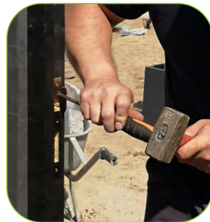
Straighten and finish up the edges of the opening.
