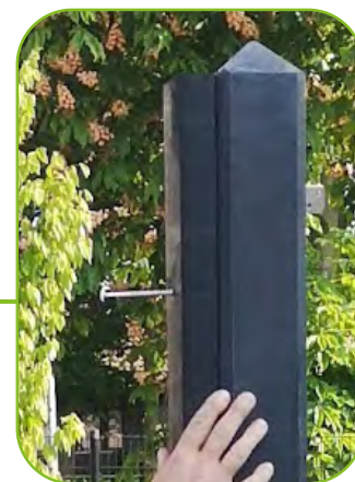
Press impact plug into holes and tighten.
