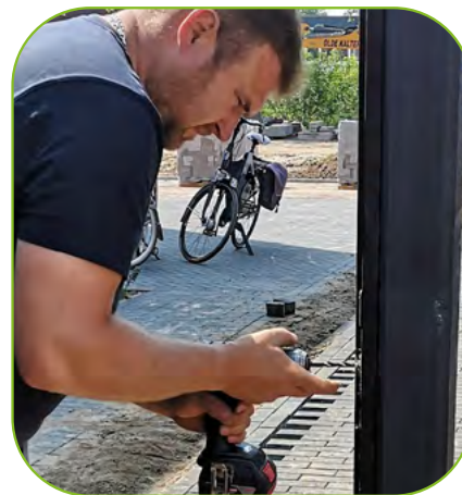
Roughly drill holes to make an opening.
